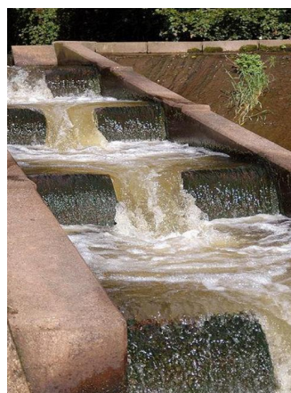
A small fish pass on the River Otter in the UK.
