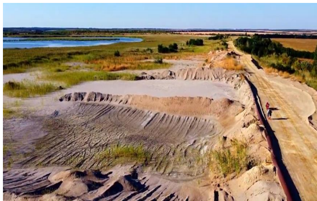
Fig. 2. Takyr and aeolian formations resembling arid morphosculpture arise with the drying of the solid phase of the tailings.
